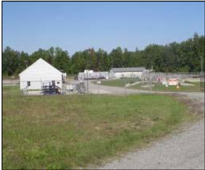
Caroline County Wastewater Treatment Facility on Rogers Clark Blvd
