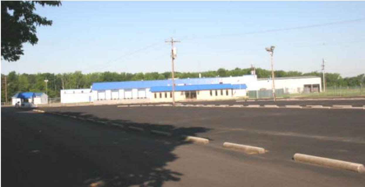
Security fence and guard house with employee parking outside the perimeter.
